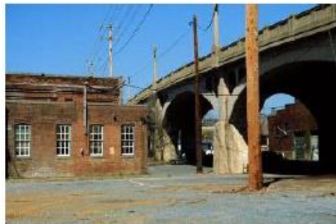
Under the Bridge, or "Retro" character of the Crossing Area
